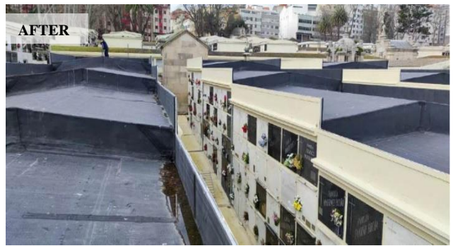
NEW ROOF INSULATION
