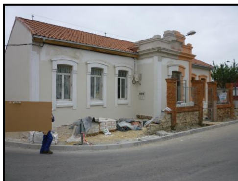
During construction works
