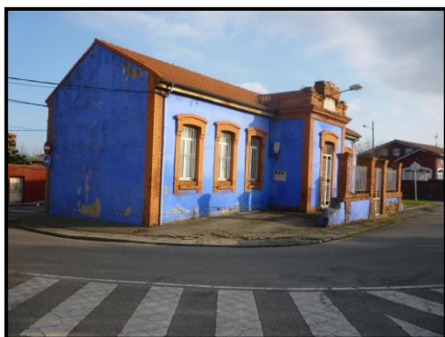
The building before de rehabilitation
