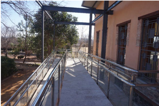
Main entrance access ramp.
