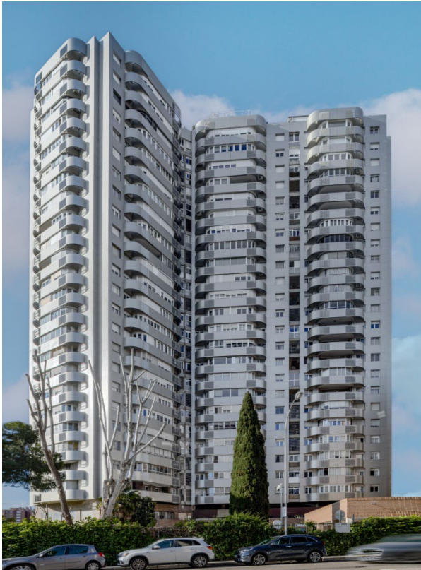
Condado de Treviño 2 building, after refurbishment. Source IDAE
