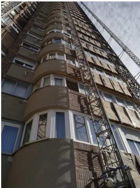
Façade renovation. Photo courtesy of Estudio de Arquitectura De Lapuerta+Campo
