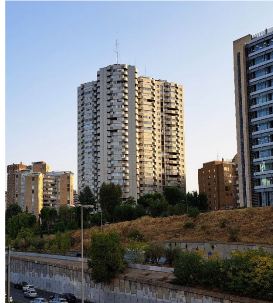
Image of Condado de Treviño building after rehabilitation. Source: Photo IDAE.
