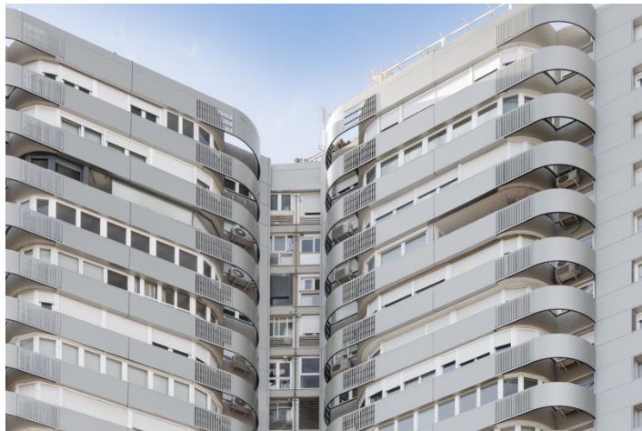
New building façade with integration of the outdoor air-conditioning units. Photo IDAE
