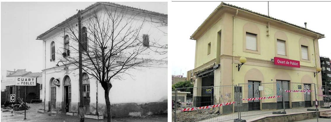
HISTORICAL PHOTO OF THE STATION / PICTURE BEFORE THE REHABILITATION
