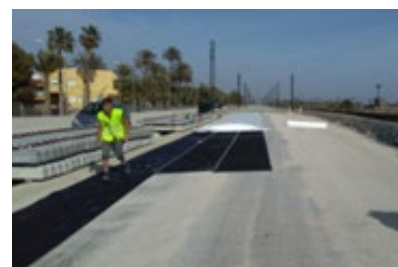
Elastomeric blanket installation at San Isidro station
