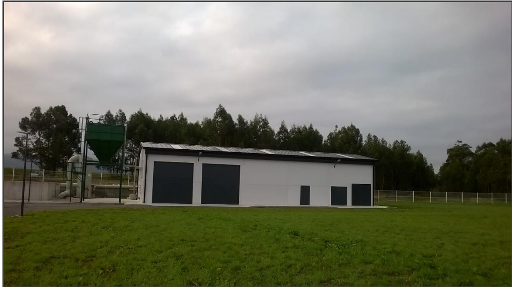
Front view from the sludge treatment building
