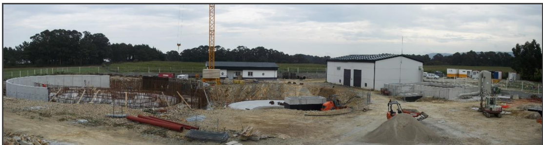
Biological Reactor and Secondary Decanting Execution Panoramic view
