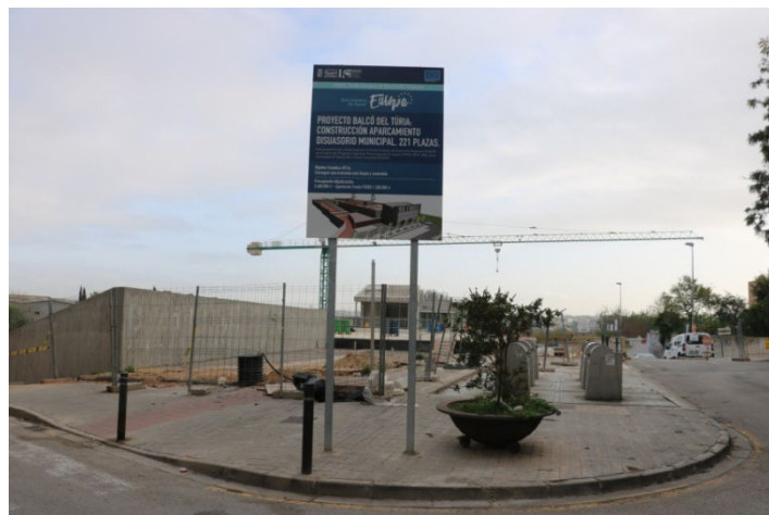
SIGN AT THE WORKS
