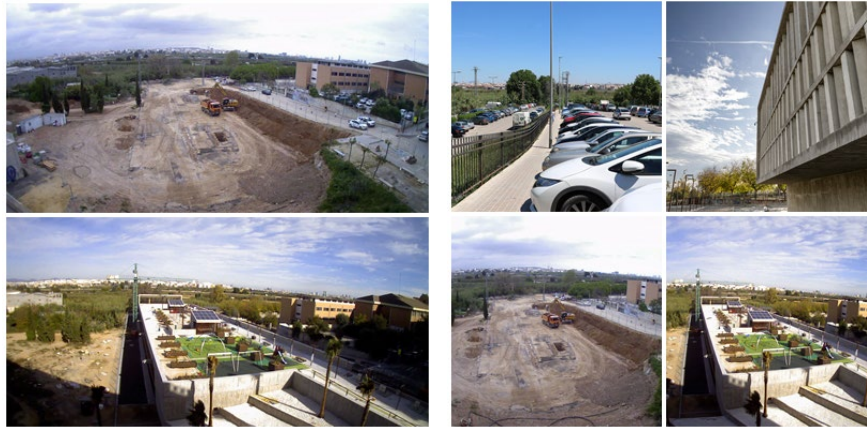
BEFORE AND AFTER PHOTOS OF THE AREA
