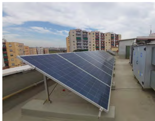
Solar panels installed on the roof
