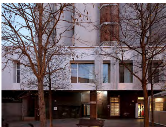
New façade of the Civic Centre rehabilitated
