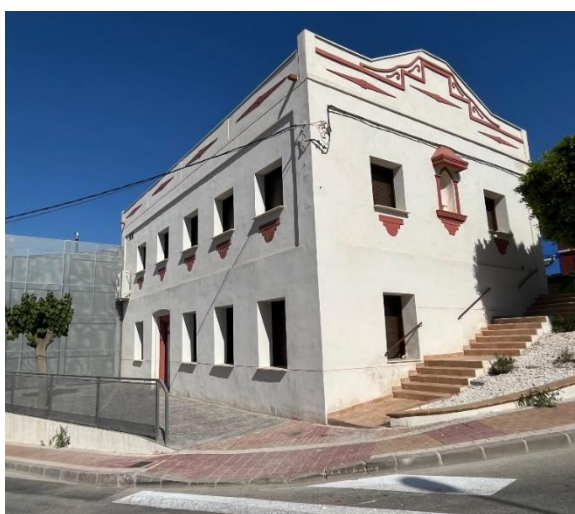
Picture of Torrealta Cultural Centre
