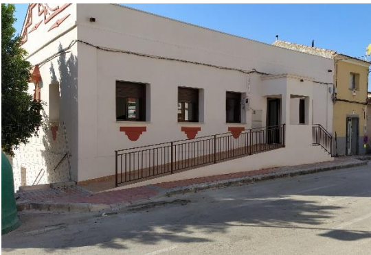
North Facade: Space ceded to the Stations of the Cross Association
