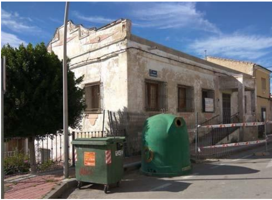
Before, North Facade
