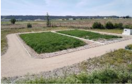
Image 1.- Esguevillas de Esgueva Wastewater Treatment Plant.
