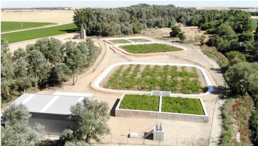
OLD FRESNO WWTP
