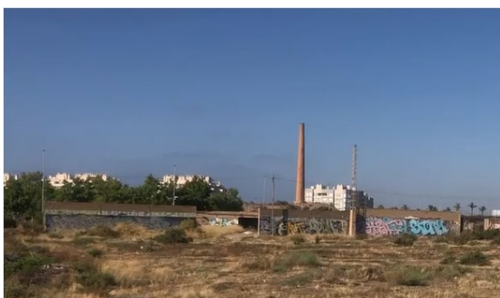
Figure 9. Space before the intervention
