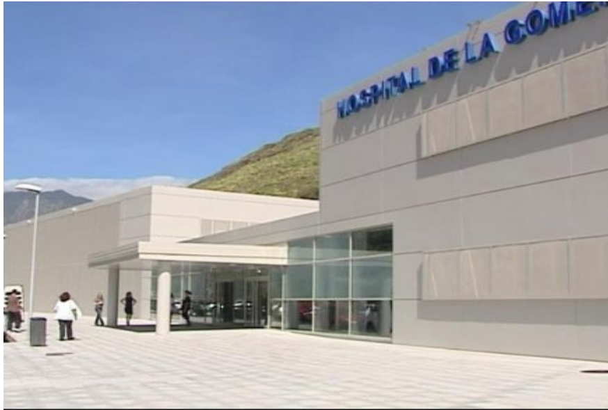
*Main entrance of the Hospital of La Gomera
