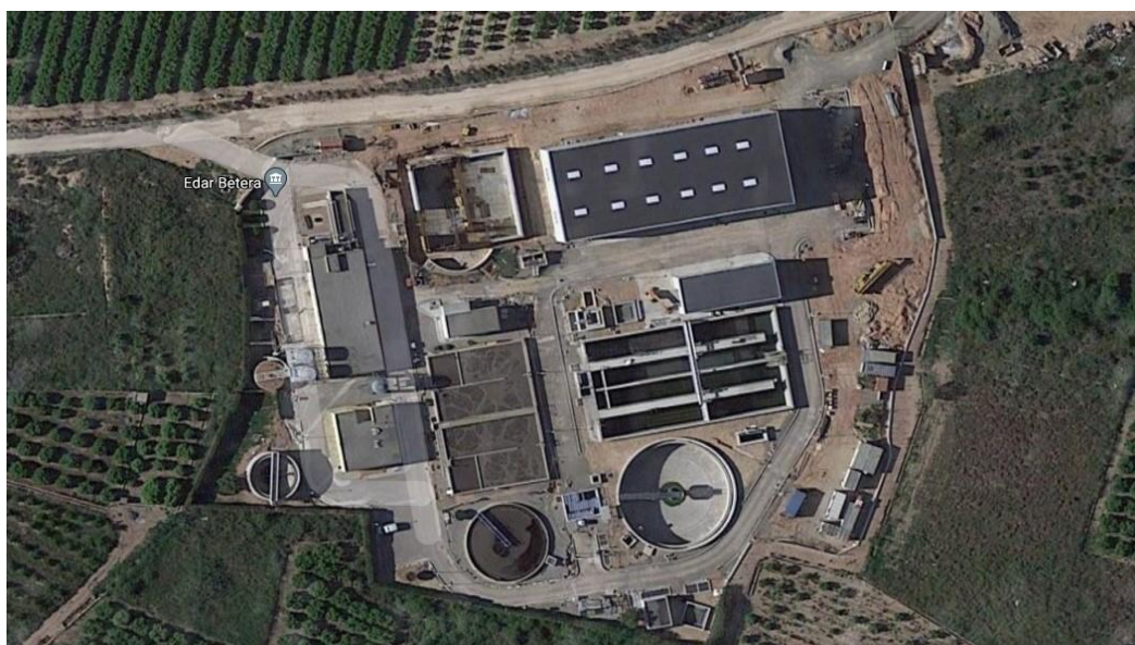
Aerial view of the station after completion of the works (November 2019)
