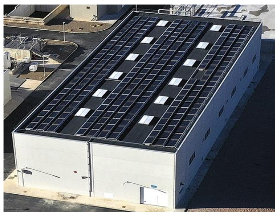
Photovoltaic installation located in the new building
