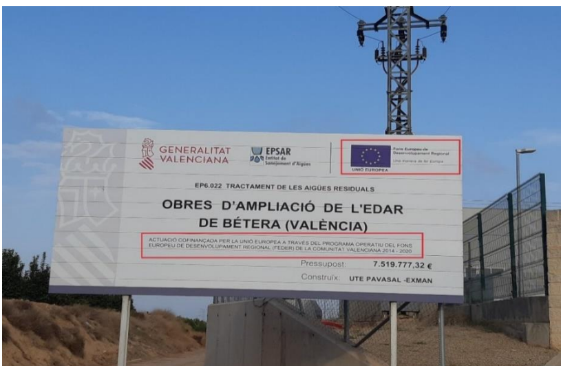
Poster at the entrance to the treatment plant during the construction of the works
