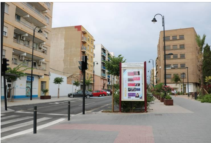
VIEW OF THE COMPLETED INTERVENTION
