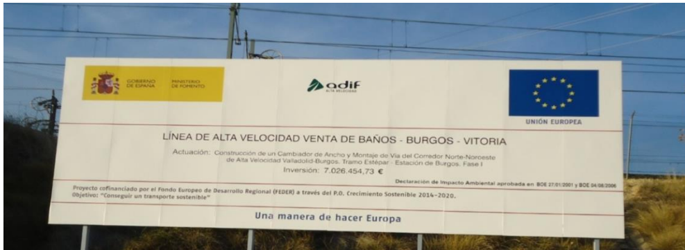
Billboard installed on the Estépar-Burgos Station section
