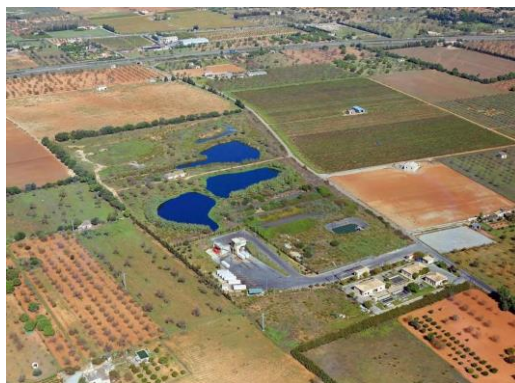
Aerial image of the Binissalem treatment plant
