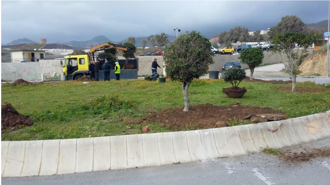
Setting up the green area
